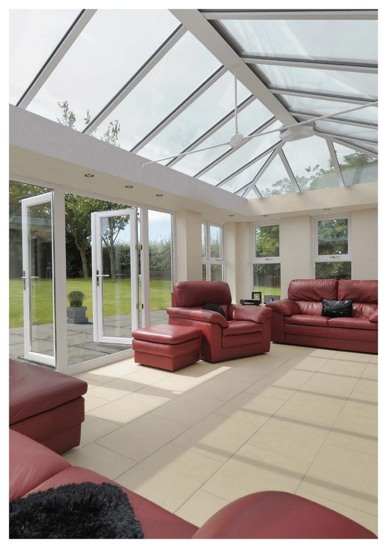
Livinroom uses an Ultraframe Classic glazed roof to which is attached a steel work ladder system at eaves and glazing bar positions. This is then plasterboarded and plaster skimmed to form a perimeter ceiling.
